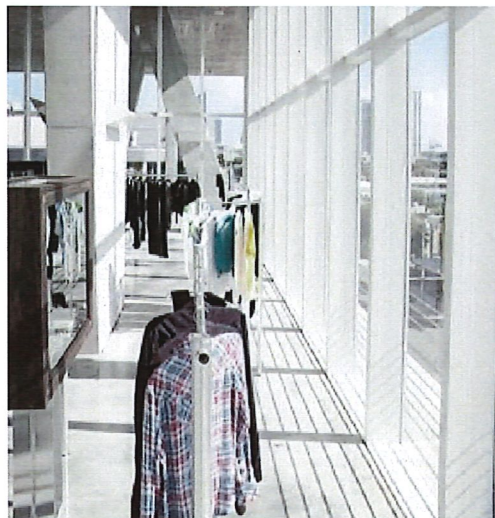
Semi-frameless glass shopfront with glazed entry doors
